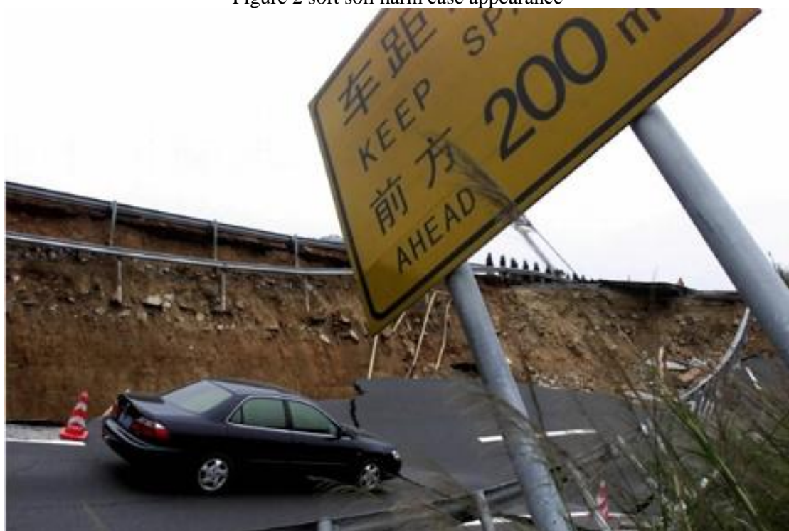
Figure 3 soft soil harm case appearance
